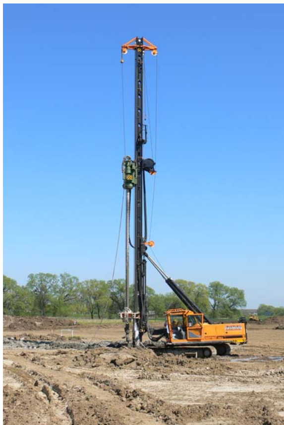
Kolumny DSM-wet [A1, Rusocin - Stabilator]
