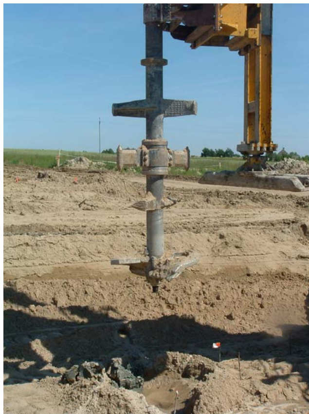
Kolumny DSM-wet [A1, Rusocin - Stabilator]
